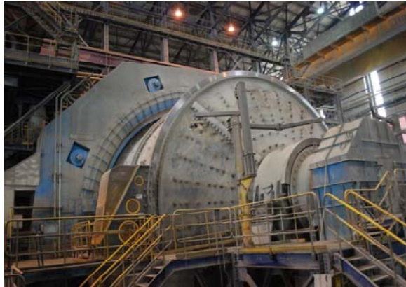
Fig. 2. Synchronous motor drive in SAG mills at copper industry.
